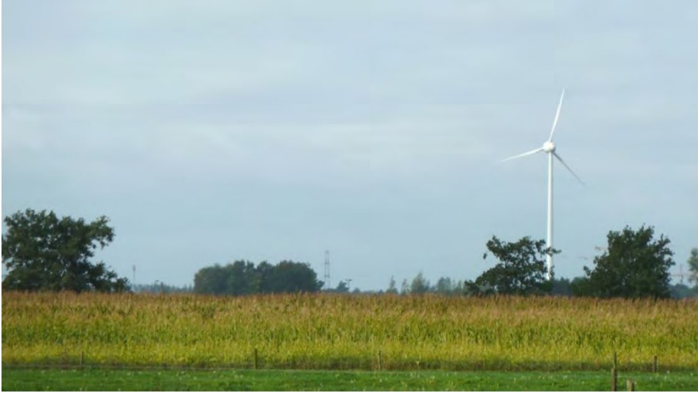
Project-MER windturbines Maldegem-Eeklo Definitief MER
